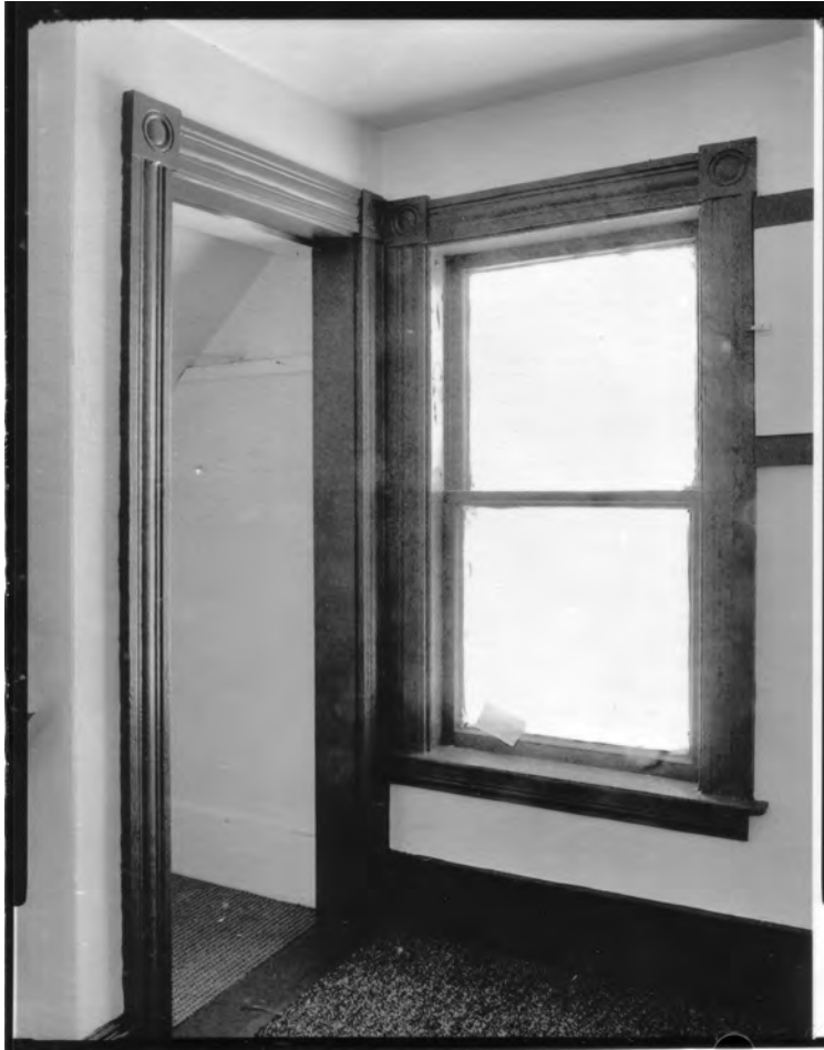
Photo 28) Attic room, showing detail of closet and front window with bullet-block trim Direction W
