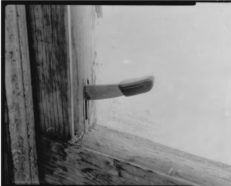
Photo 23) Dining Room, detail of window hardware on 1/1 sash window; this hardware found on most windows on second floor Direction: W
