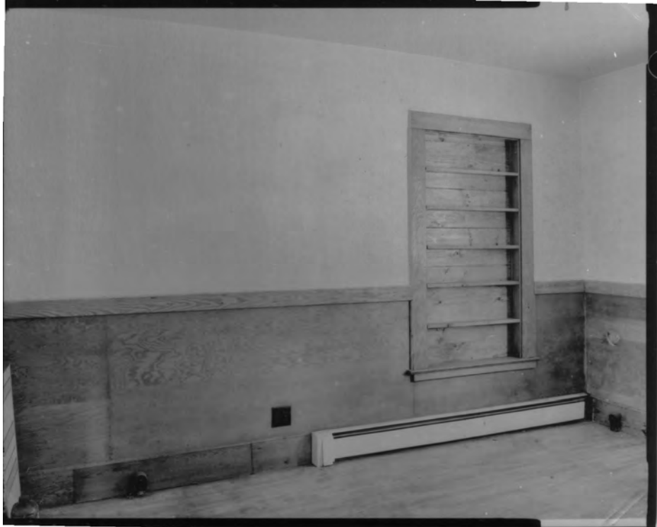
Photo 9) Dining room/kitchen, showing original blocked window in cross-gable section, and later wainscoting Direction: S
