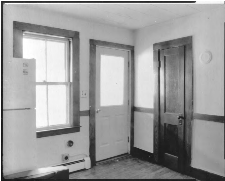
Photo 16) Kitchen, showing only remaining 2/2 sash window, entry, closet, and thimble in original stove-flue chimney Direction: W
