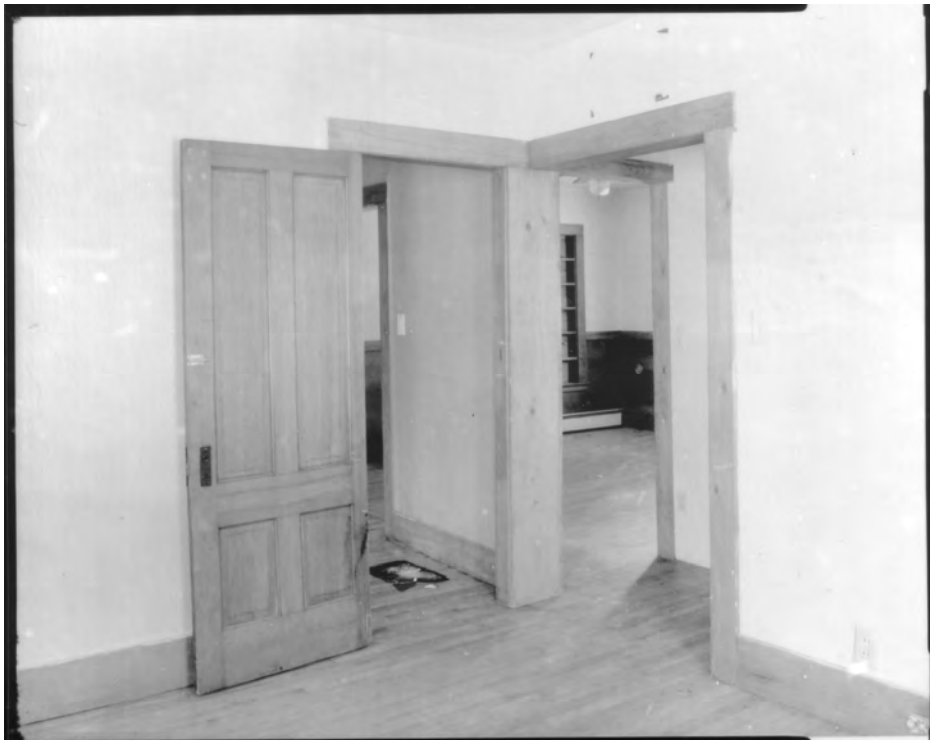
Photo 12) Northwest room, show doorway to northeast room with original four-panel door with original hardware and added or altered doorway to small hall Direction: S
