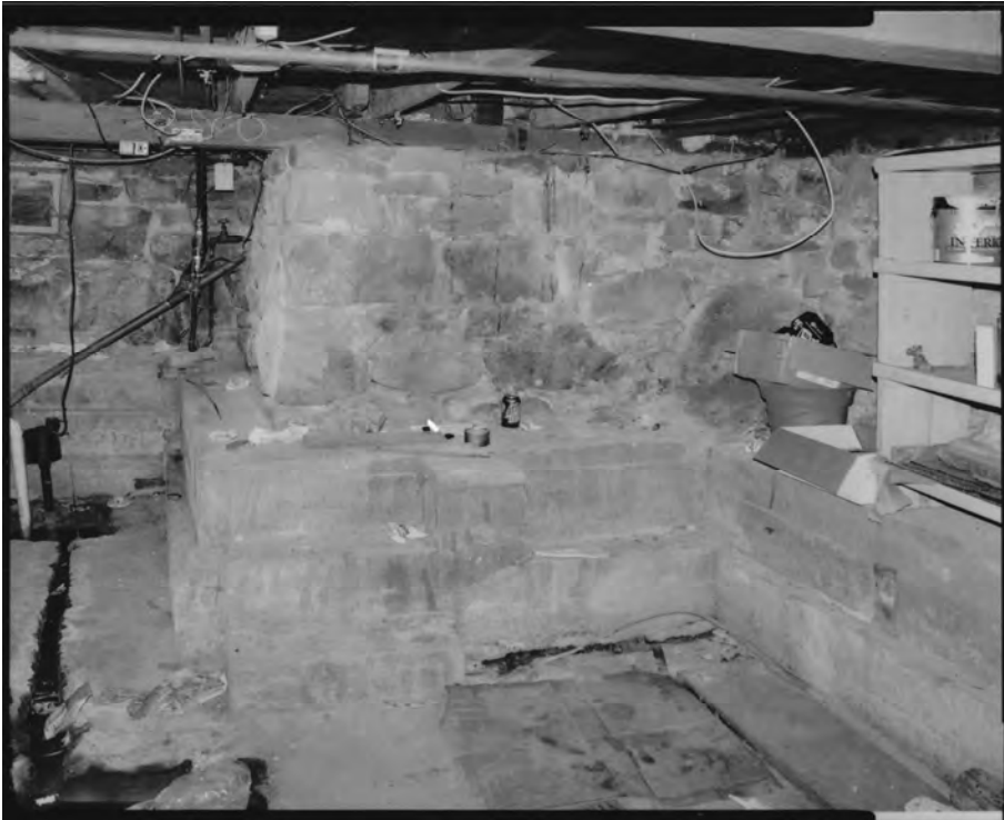
Photo 7) Stone foundation and poured concrete form work at intersection of cross-gable and main block Direction: SW
