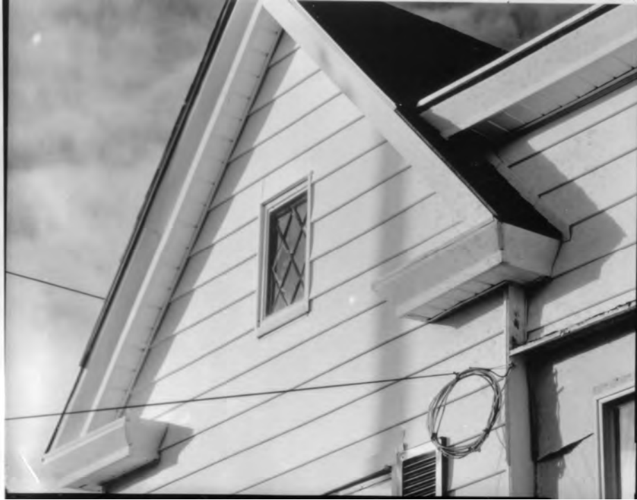
Photo 6) Detail, gable end of cross-gable with diamond pane window, raking cornice, and cornice returns Direction: N
