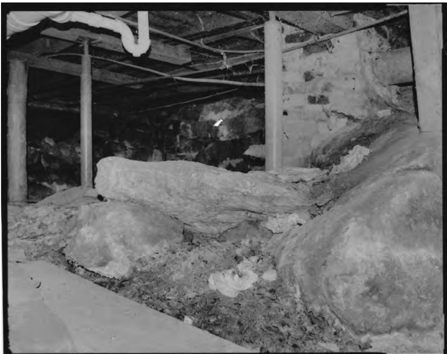
Photo 8) Crawl space under rear ell, showing base of stove-flue chimney atop a ledge Direction: SE
