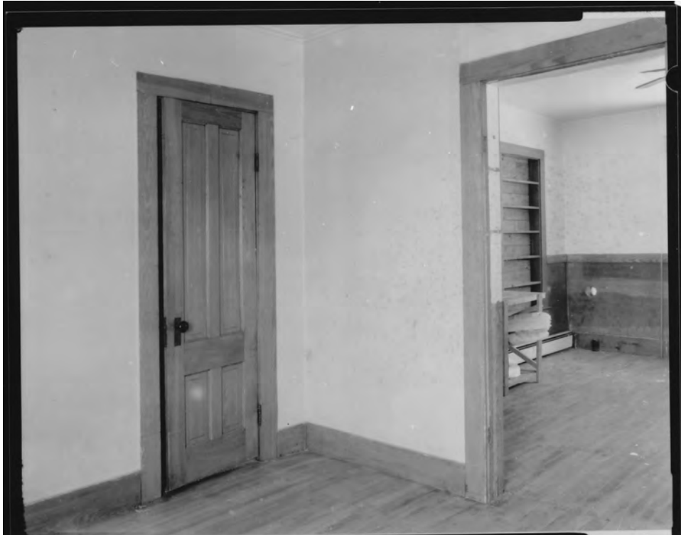
Photo 13) Northeast room, closet with original four-panel door and hardware and doorway to dining room/kitchen Direction S
