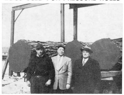
The huge logs pictured above arrived recently from Rutland, Vermont, and are to be converted into pressrolls at the Cascade plant for use on some of our paper machines. They are all Vermont Rock Maples with the longest one (on the left) tipping the scales at 8,000 pounds. Also pictured, left to right, are the truck driver, (unidentified), Lewis Blanchard, and Perley R. Eaton, Rutland, Vt.
