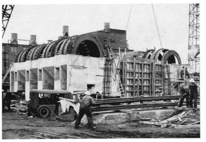
Work progresses on Barking Drum: Three new barking drums are to be installed in a new, modern building which will be constructed north of the present Barking plant. The plant will operate in conjunction with the new unloading conveyor which is designed to accommodate many more cords of wood regardless of whether they arrive via rail or truck.
