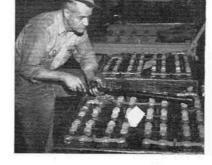
Shown adding distilled water to one of the batteries used by the electric trucks at Cascade is Arthur Wentworth, a 14-year man.
