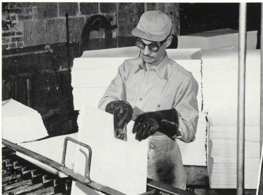
STEEPING AND SHREDDING . . . First step in converting Brown Company pulp to cellophane is soaking in caustic soda (above). The moist pulp is shredded into crumbs, placed in steel containers to age and then mixed with chemicals (right).
