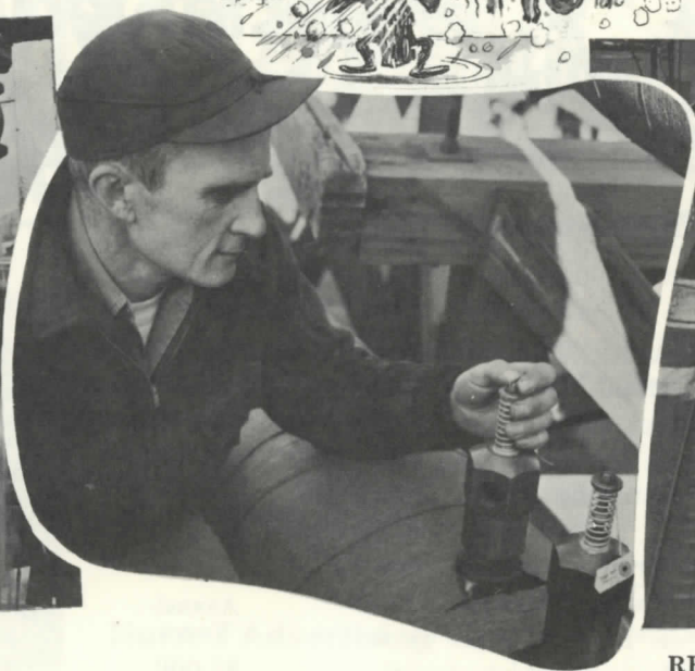
VACUUM BREAKERS . . . Piper Leader Norman Farrington examines vacuum breakers installed at high points in line to prevent any possible damage or collapse when line is drained.
