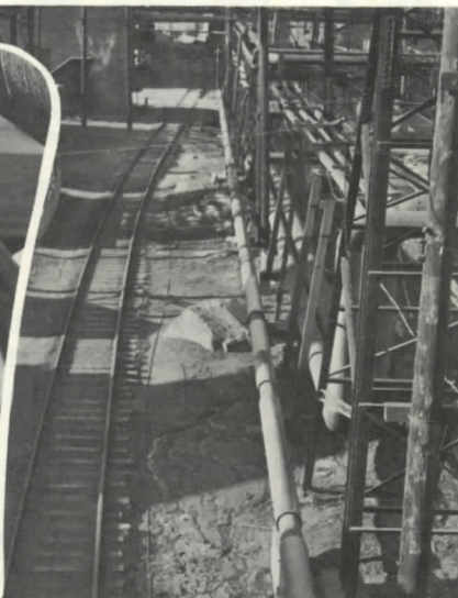
READY FOR TESTING . . . Section of new 1,100 ft. pipe line between Sulphite Washers and Debarking Plant. 14 in. pipe is insulated except at joints, which will be covered after line is tested for leaks.
