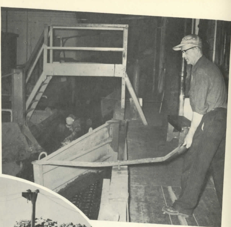
Ephraim Lamontagne, at entrance to barking plant, controls flow of wood into three drums using steel gate to spill wood from conveyer into drum.
