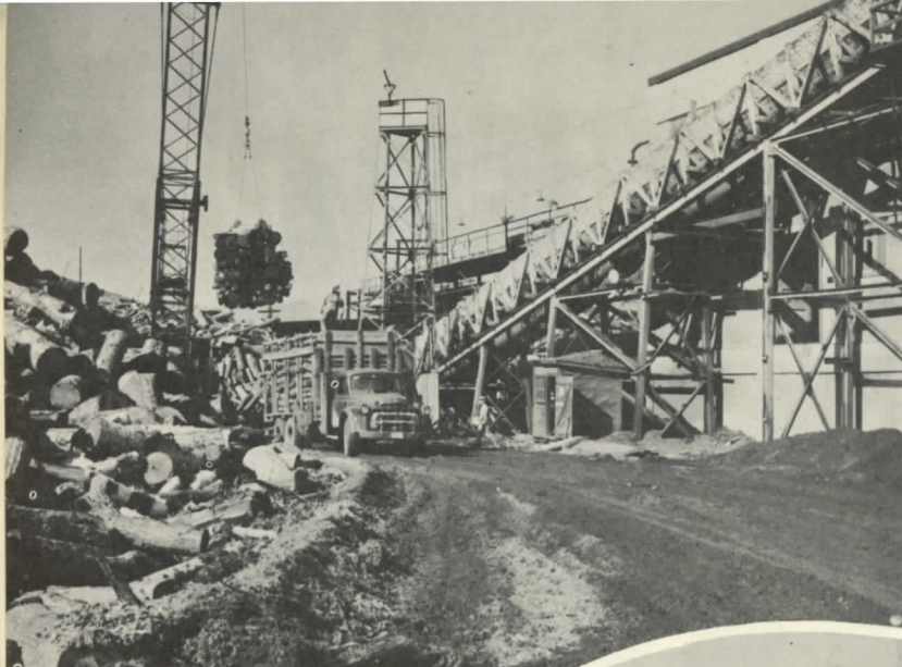
Crane unloads hardwood, full tier at a time, tosses it into storage pile or conveyer, depending on mill requirements.
