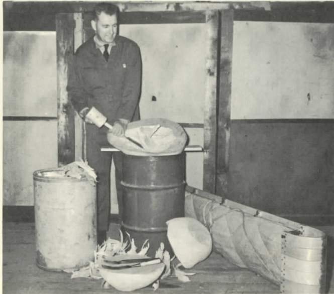
CHISELING OUT BURL . . . After burl is shaped on outside, tedious job of hollowing out center begins. Gus Korn has also made two toboggans in home workshop, and carriers for top of car.
