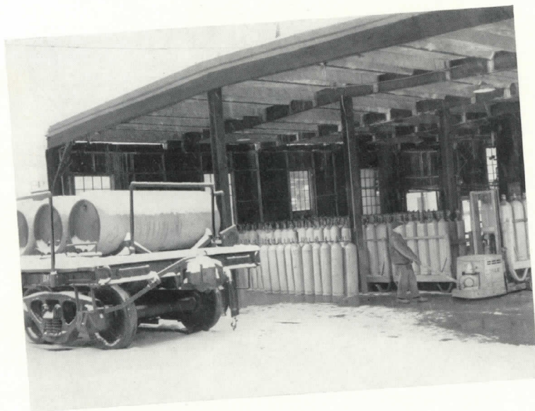
12. Chlorine is shipped in these two types of cylinders and is used for water purification.
