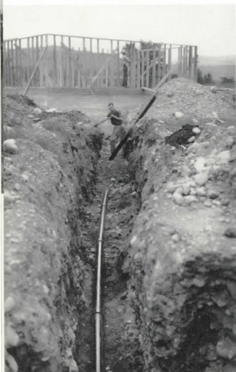
19. Sewer pipe installation at Bud Potter's home in Berlin.
