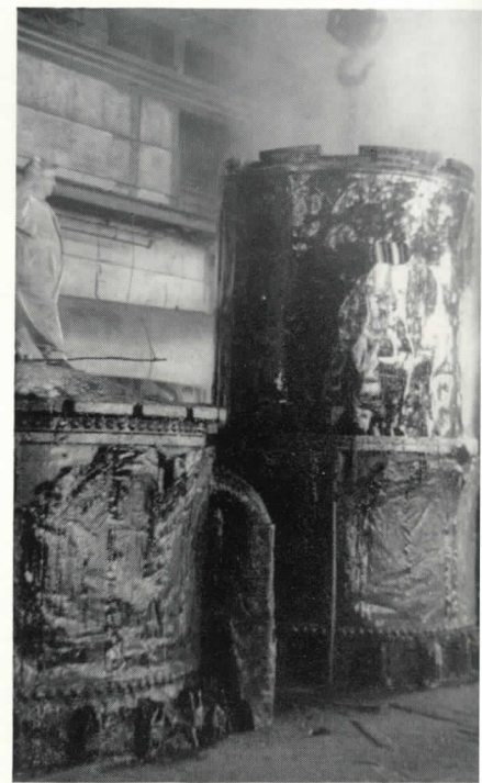
8. Emery Moreau, plugman, directs crane in raising tank after treating.
