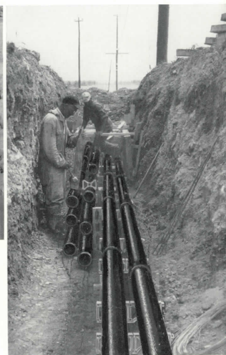
21. Bermico electrical conduit installation using plastic spacers.
