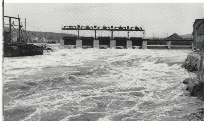
Water was at highest point at 3:30 p. m., April 23 when all 5 gates were opened to allow 14,500 cu. ft. of water per sec. to flow through gates. Note that water is not overflowing gravity section of dam at right.
