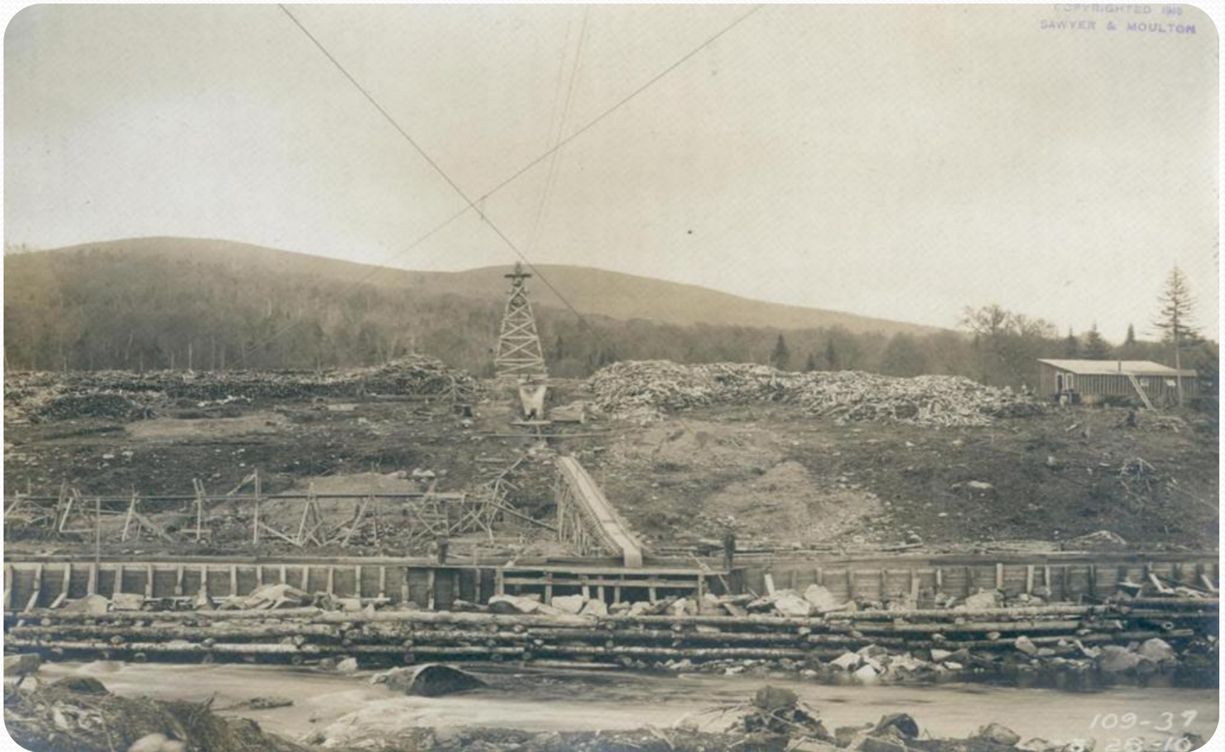
View near station 'D' looking south into core wall trench Sluicing Giant in operation (May 28, 1910)
