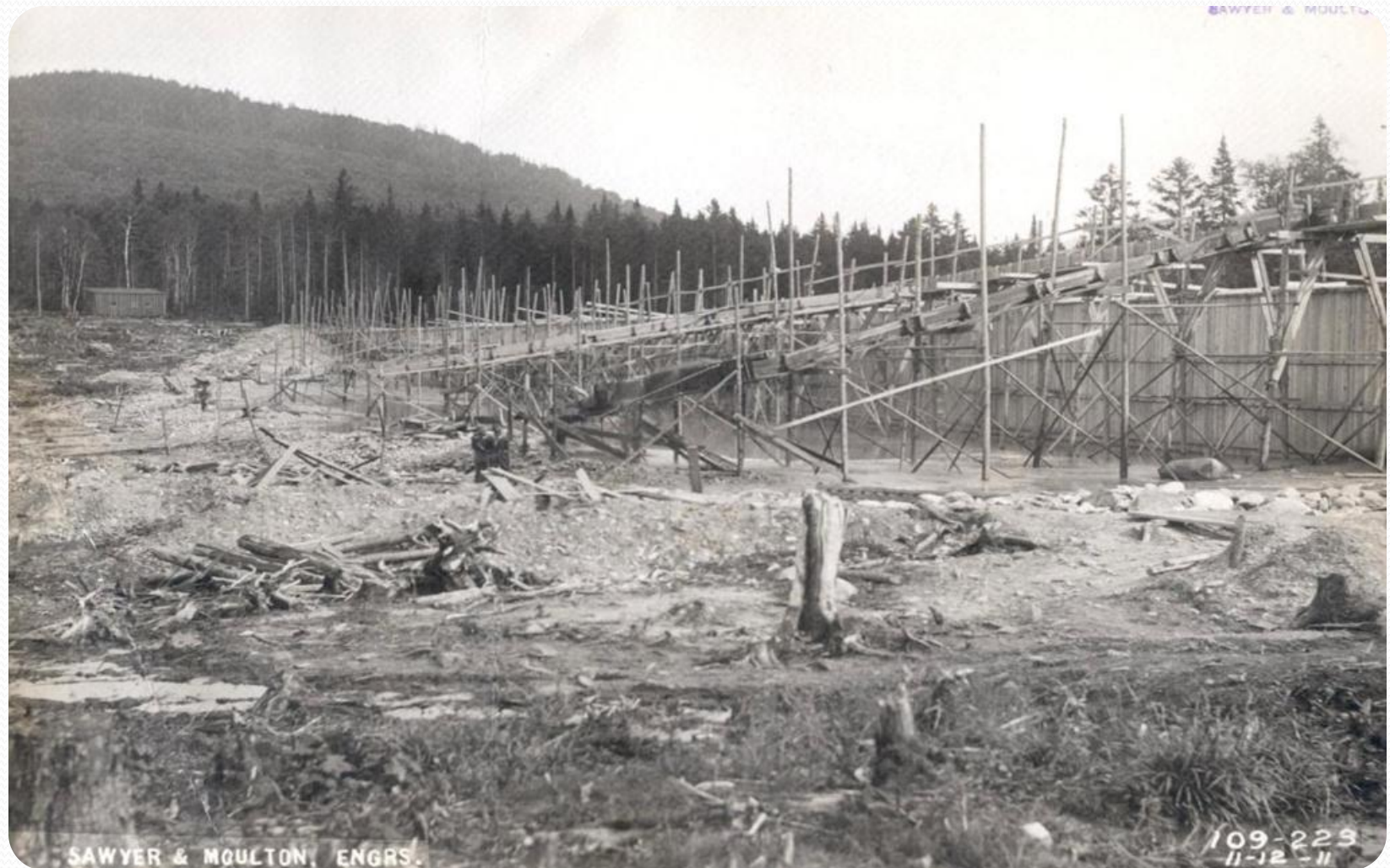
Filling east side of Abbott Brook dike November 12, 1911
