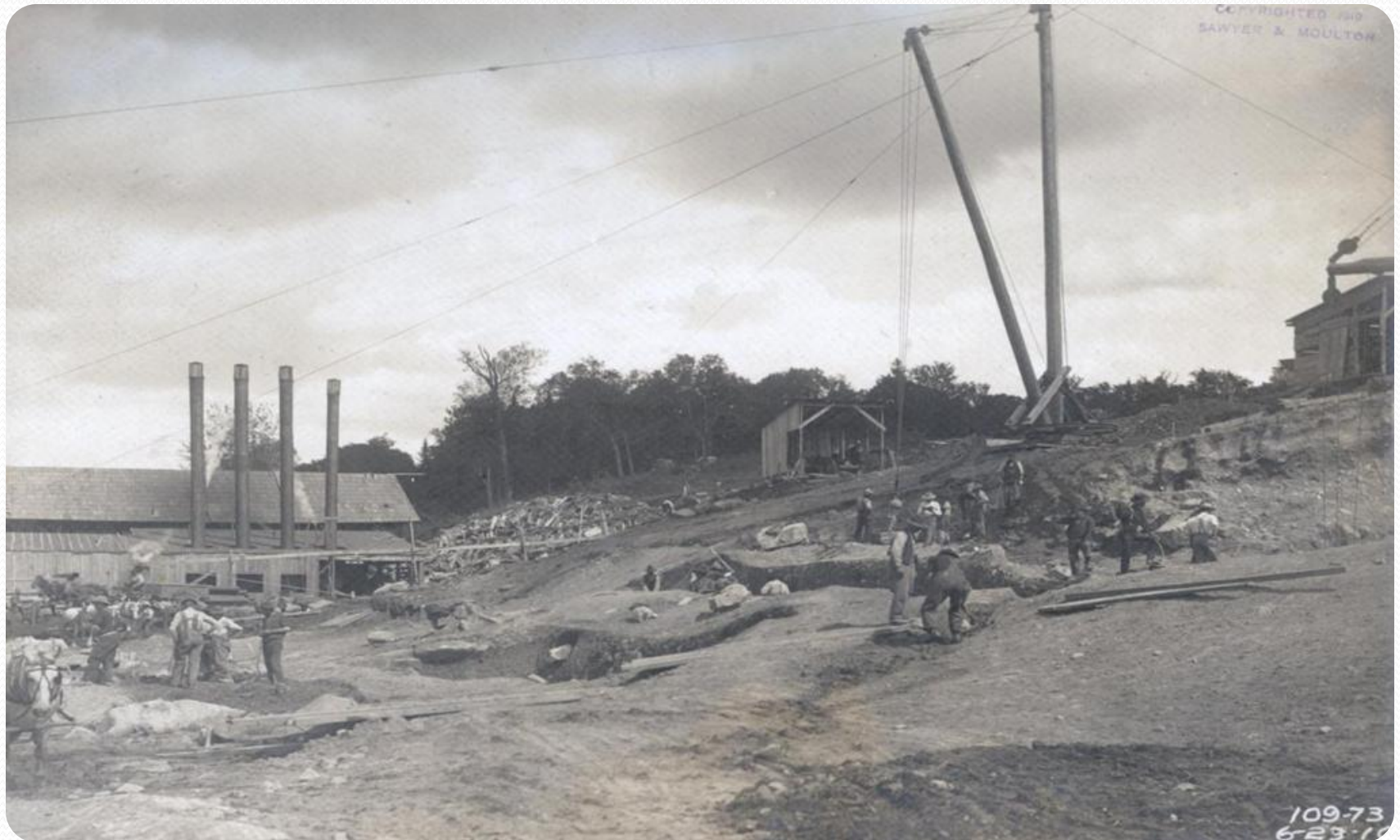
View near station 'K' looking southeast at excavation for buttress No.1 Old dam and boiler house No. 2 in background June 23, 1910
