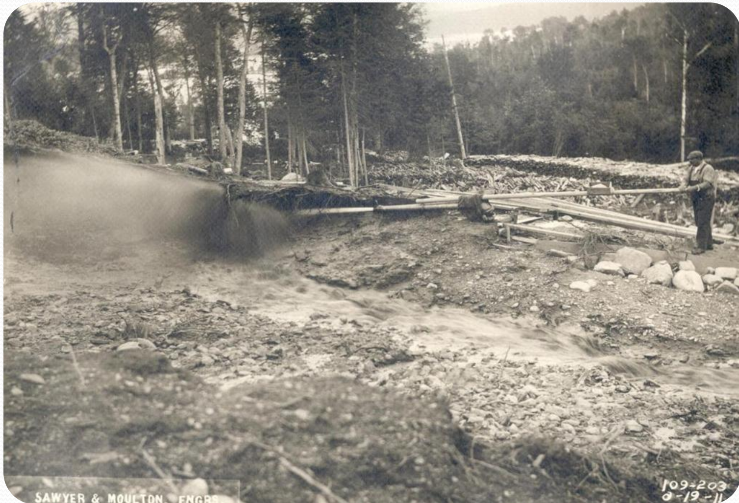
Abbot Brook dike; hydraulic giant in foreground, new lake in background June 19, 1911
