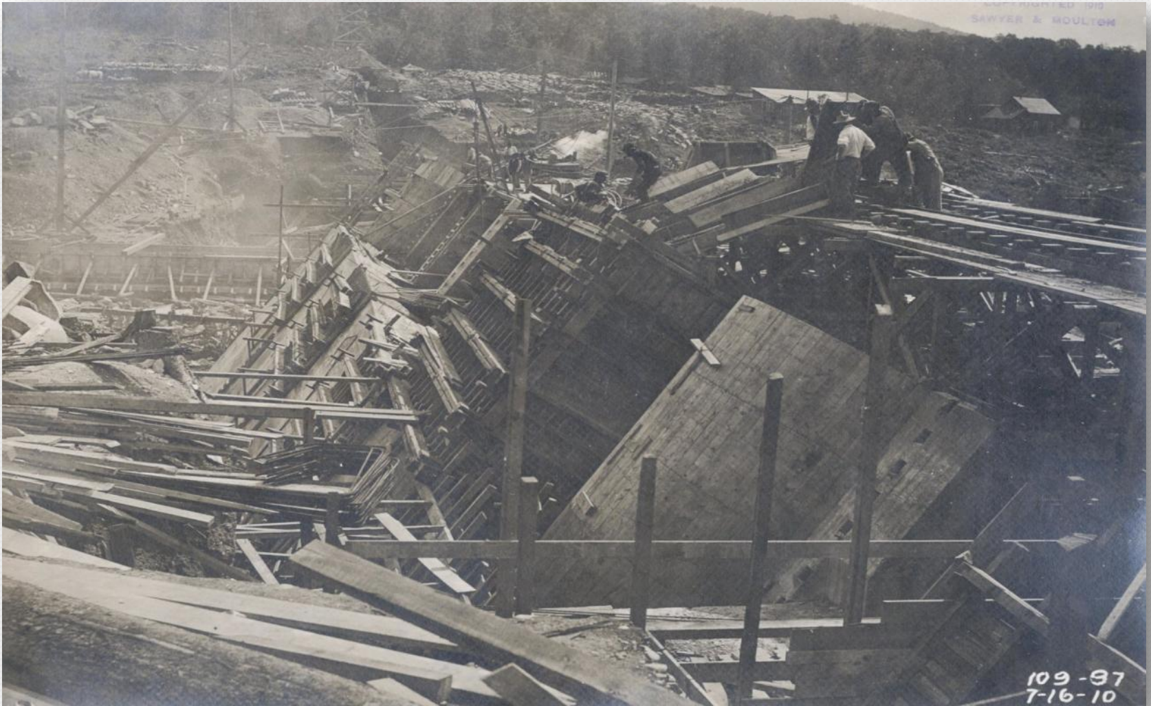
View looking south along face of spillway Placing concrete from tracks July 16, 1910
