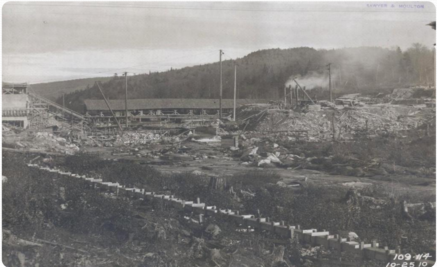
Looking upstream toward dam construction, spillway at left October 25, 1910
