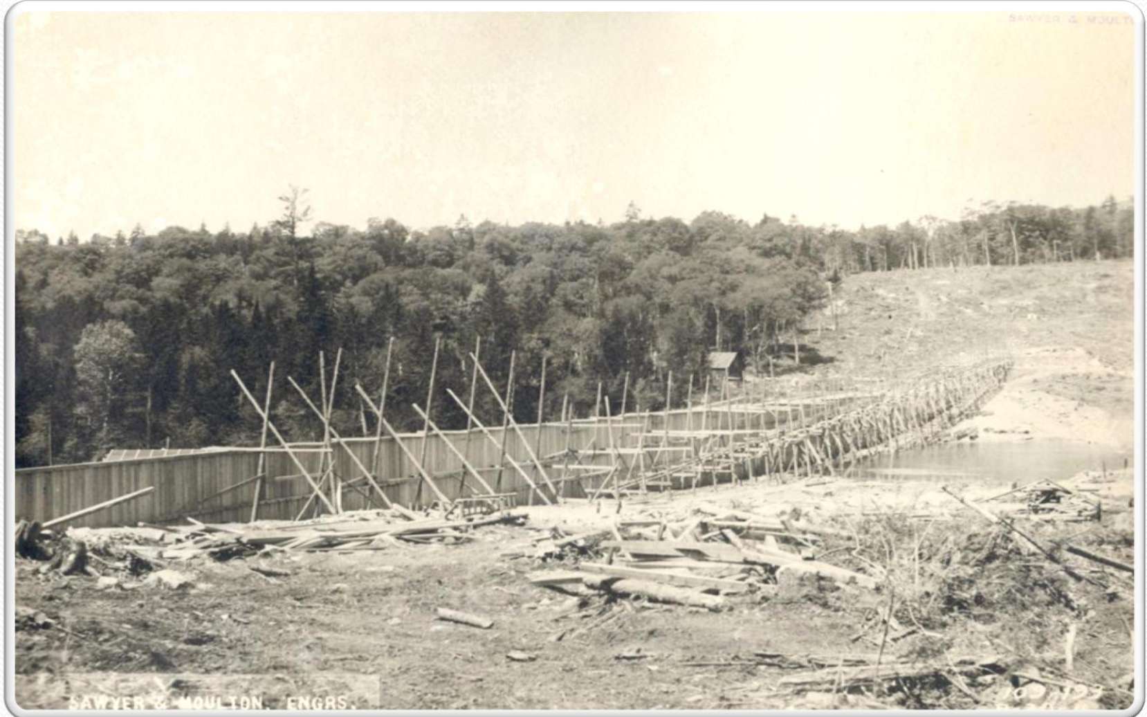
Abbott Brook dike looking northwest at core piling and sluicing trestle May 30, 1911
