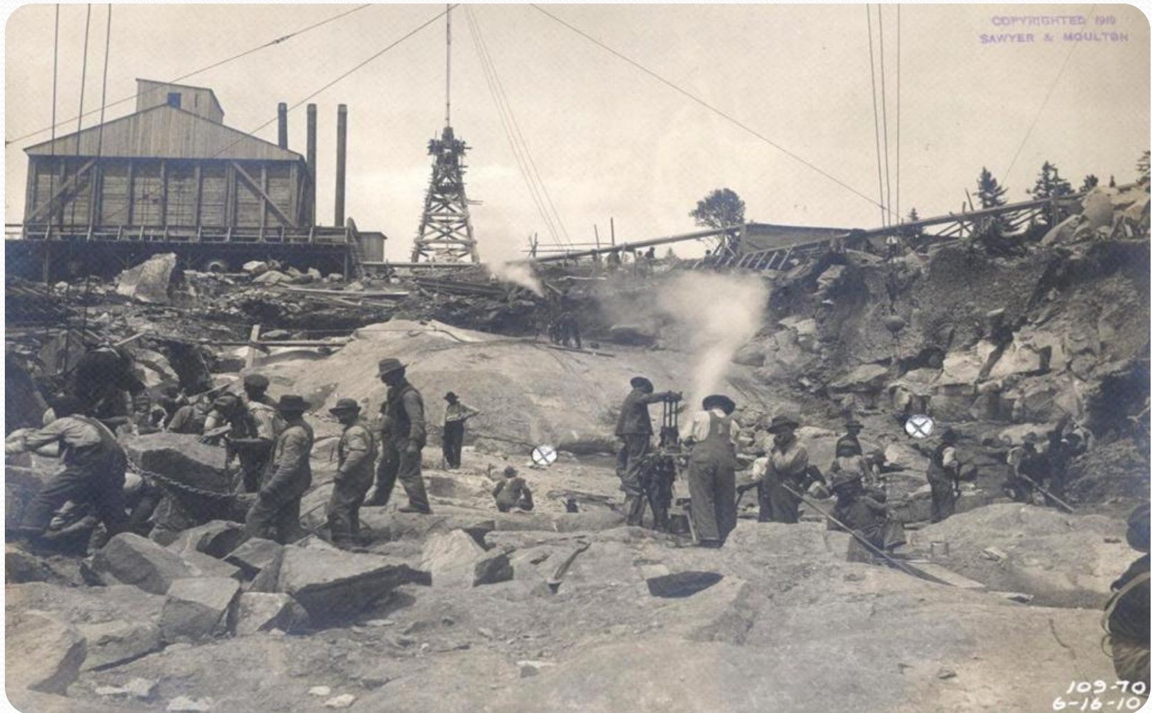
View east of station 'J' looking north at spillway excavation. Crosses indicate seams of rotten ledge underlying sound ledge June 16, 1910
