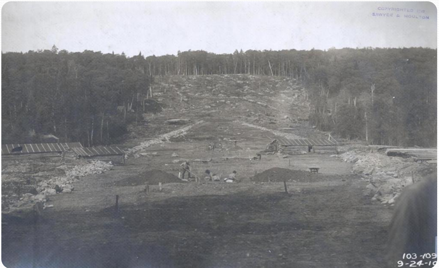
View on center line of Abbott Brook dike looking north Grubbing completed September 24, 1910
