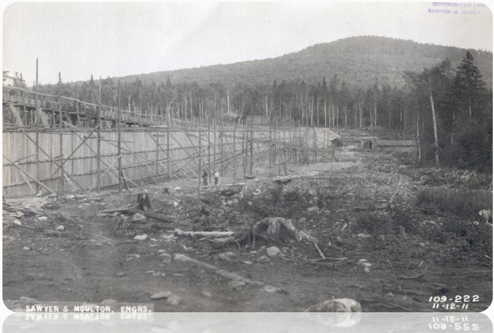
Filling west side of Abbott Brook dike November 12, 1911
