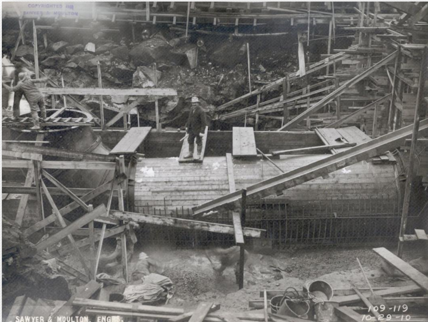
North outlet tube set, concrete being placed October 29, 1910
